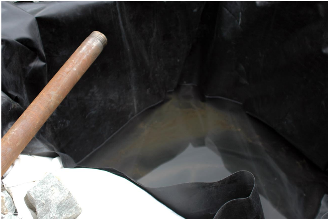
PHOTO 9: An empty mud settling pond
