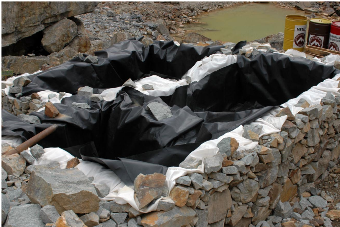
PHOTO 8: The mud settling ponds with impermeable membrane
