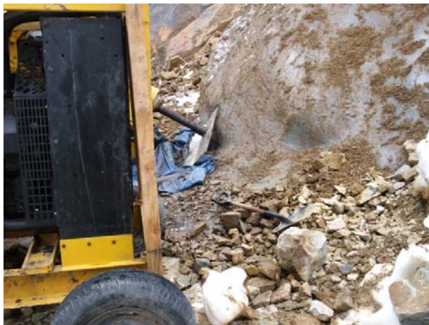
An exploration drill obviously perforating the glacier. WGS84 UTM Zone 18s 282555E 8861436N –altitud 4848. Date: March 29 2011. Photo: Marco Arenas.
